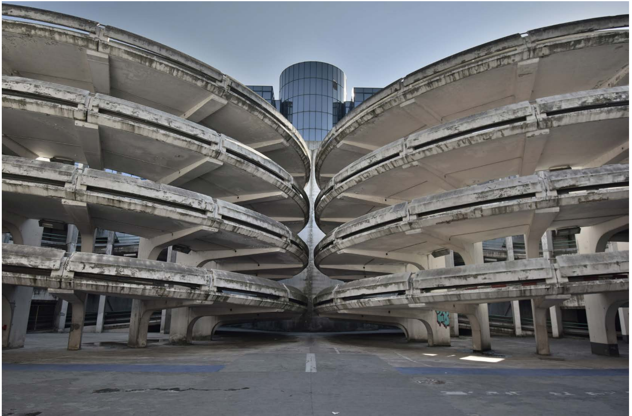
Le parking Silo
